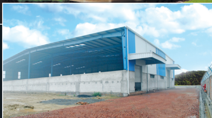
Tyre Plant Under Construction at Sonipat Haryana
